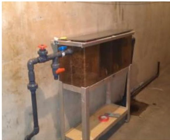
Figure 5. Biobox (treated) at the Outlet of the Treated System.
